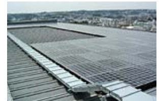
■ Yokohama Office (58kW) (introduced in FY2012)
