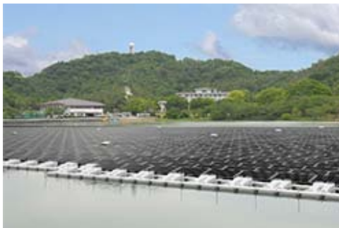
Sakasamaike Floating Mega Solar Power Plant (approx. 2.3MW, operation started in June 2015), Hyogo Prefecture
