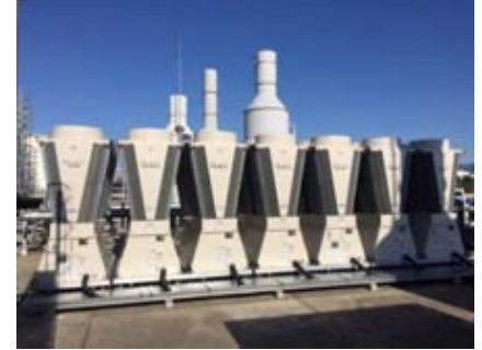
High-efficiency heat pump chiller
