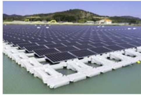
Takaoka Nishi Floating Mega Solar Power Plant (approx. 1.7MW, operation started in March 2015), Hyogo Prefecture
