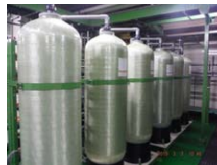
Wastewater recycling equipment
