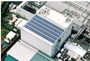
■ Kagoshima Hayato Plant (40kW) (introduced in FY2006)
