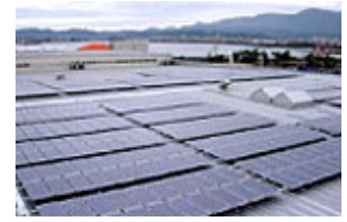
■ Mie Ise Plant (366kW) (introduced in FY2005 and expanded in FY2016)
