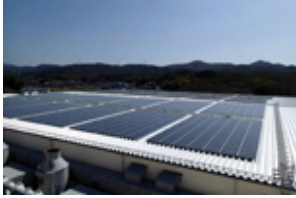
■ Kyoto Ayabe Plant (1,500kW) (introduced in FY2014 and expanded in FY2016)
