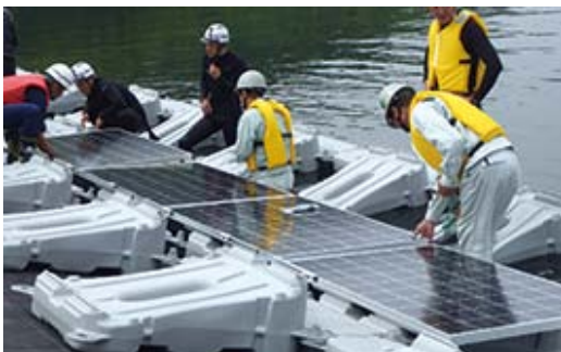
Floating platforms being installed on the water
