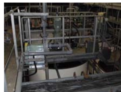
Effluent treatment plant
