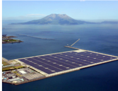
Kagoshima Nanatsujima Mega Solar Power Plant where the Solar Science Museum is located
