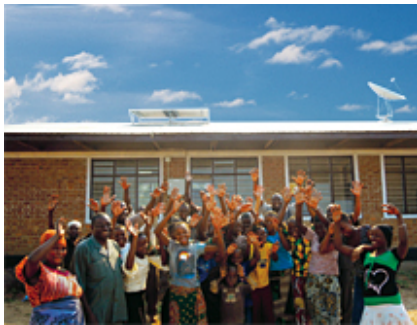
Solar modules installed at a school (Tanzania)
