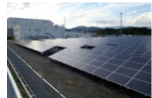
■ Fukushima Koriyama Plant (1,500kW) (installed in FY2014)
