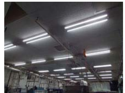
LED lights installed at Kagoshima Kokubu Plant
