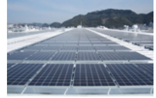
■ Kagoshima Kokubu Plant (1,100kW) (introduced in FY2006 and expanded in FY2014)
