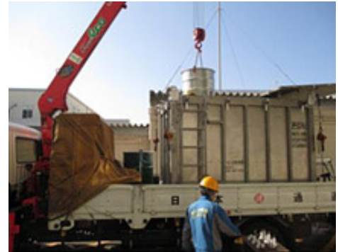
Transporting operations for outsourced disposal (Kagoshima Sendai Plant)
