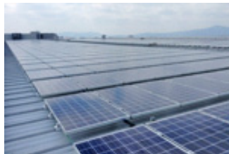
■ Shiga Yasu Plant (590 kW) (introduced in FY2011 and expanded in FY2014)
