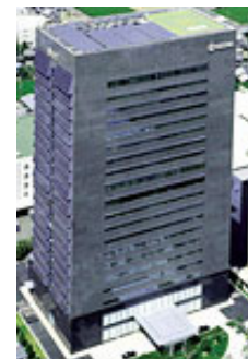
■ Head Office (214 kW) (introduced in FY1999)
