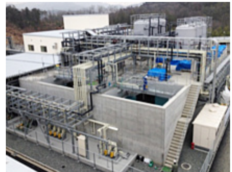
Effluent treatment equipment newly installed at Kyocera SLC Technologies Corporation's Kyoto Ayabe Plant
