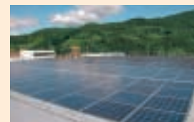
Water purification plant (Japan)
