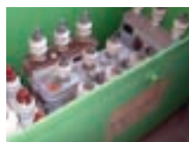
Storage of PCB wastes
