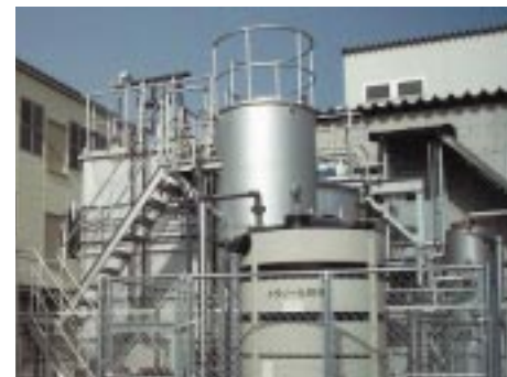
Denitrification processing facility (Shiga Yohkaichi Plantss)
