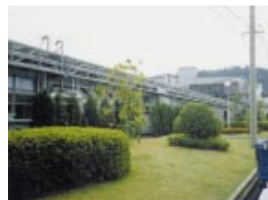
Making underground pipes aerial (Kagoshima Kokubu Plant) Aerial pipes allow for easy visual inspection.
