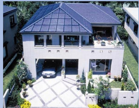
The Econoroof Solar-Powered Roof Cover (for hipped roofs)
