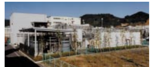
Discharged plating water processing facility (Kagoshima Kokubu Plant)
