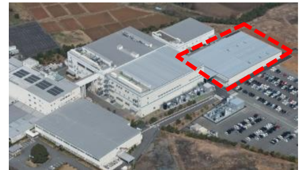
Factory No. 7 at the Tamaki Plant, Mie, of Kyocera Document Solutions Inc.
