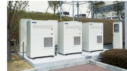
Installation of SOFC* Systems (Shiga Yohkaichi Plant, Japan) *Solid Oxide Fuel Cell
