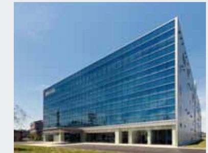
Nakayama Office (Yokohama, Japan)
