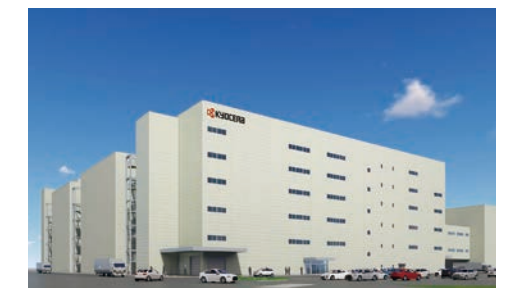
Conceptual drawing: New building at Kagoshima Sendai Factory (planned to open in March 2025)
