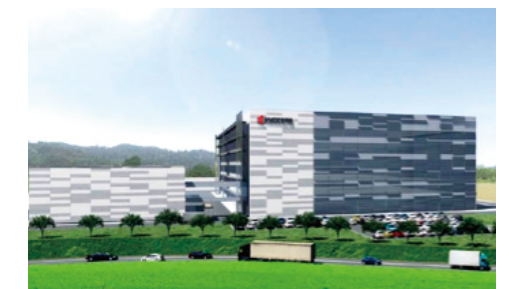
Conceptual drawing: New factory in Isahaya City, Nagasaki Prefecture (planned to open in March 2027)
