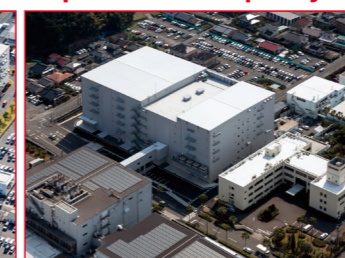
The new building at the Kagoshima Kokubu Plant
