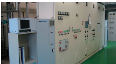
24-hour nonstop COD / cyanogens monitoring system for final effluent (Shiga Gamo Plant)
