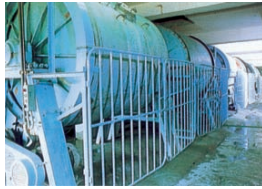
RAW MATERIAL MILLING AND MIXING
