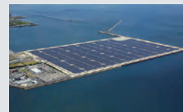
Kagoshima Nanatsujima Mega Solar Power Plant
