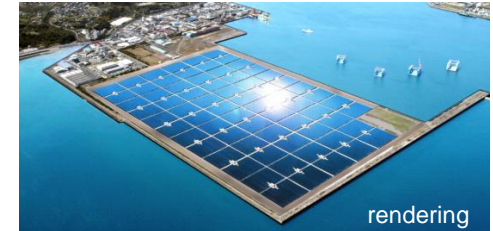
Kagoshima Nanatsujima Mega-Solar Power Plant
